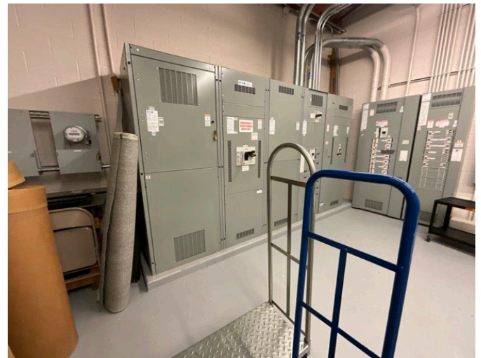
16 - SECONDARY SWITCHBOARD
